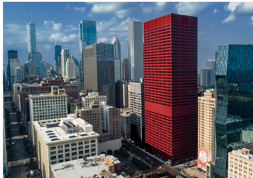
„BIG RED“ PRIME OFFICE TOWER – CHICAGO
